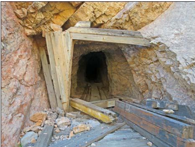
Figure 1. Azure Mine, lower Adit (view S) 2
