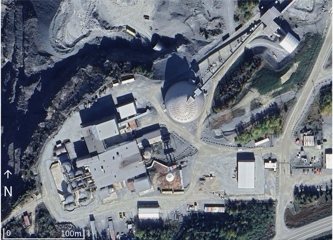
Figure 17-4: Process Plant Aerial Photo (Google Earth 2023)
