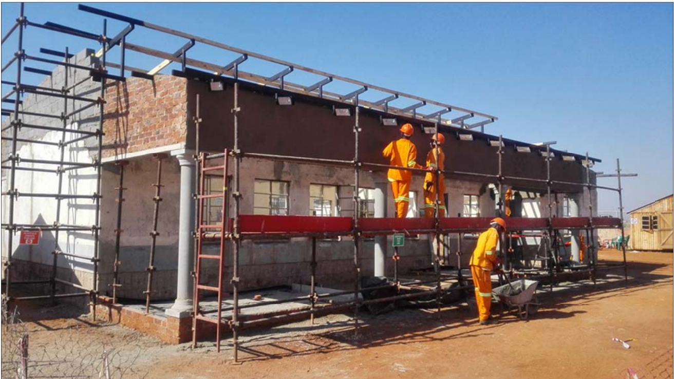
Figure 8: Renovation of a community care centre in a host village.
