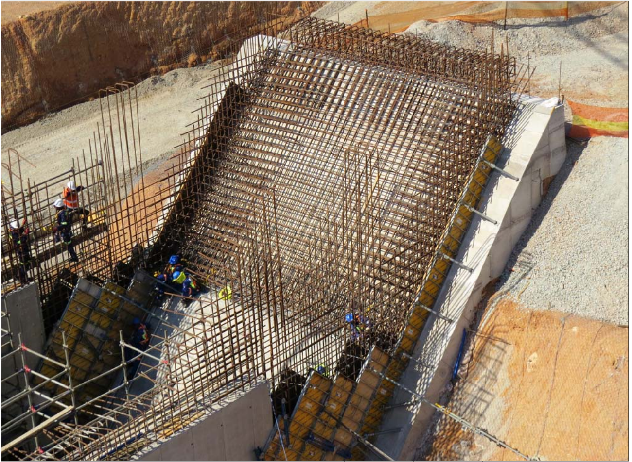
Figure 7: Construction of the lined storm-water pond.
