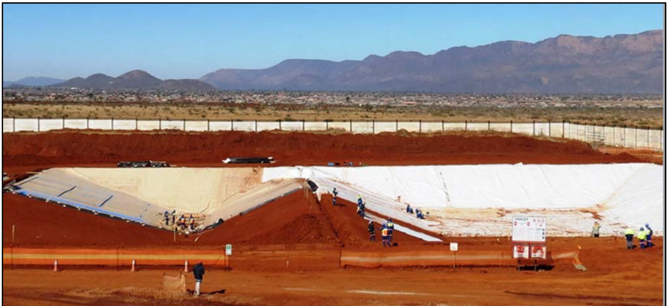
Figure 7: Construction of the lined storm-water pond.
