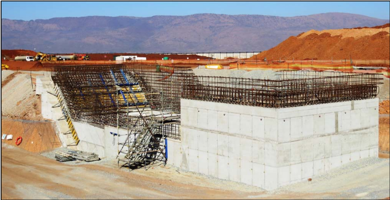
Figure 3: Shaft 1 collar and ventilation plenum construction, July 2015.
