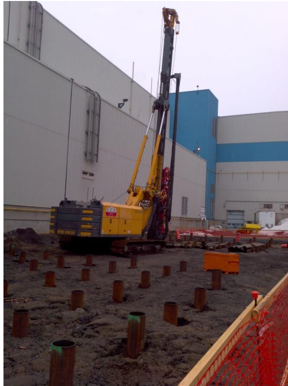
Figure 24.21 – Piling West of Building #80
