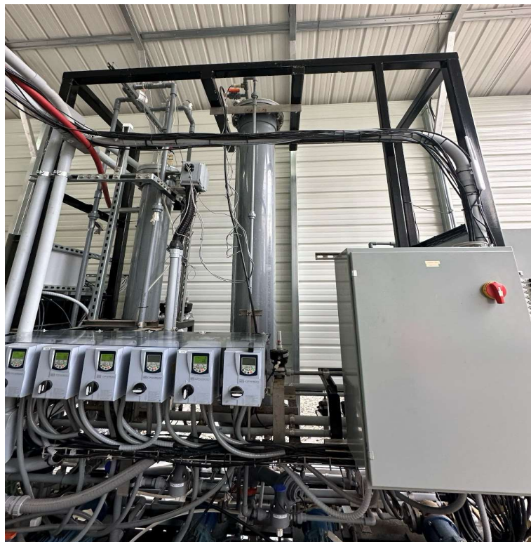
Figure 13-5: LSS Column at the Pilot Plant
