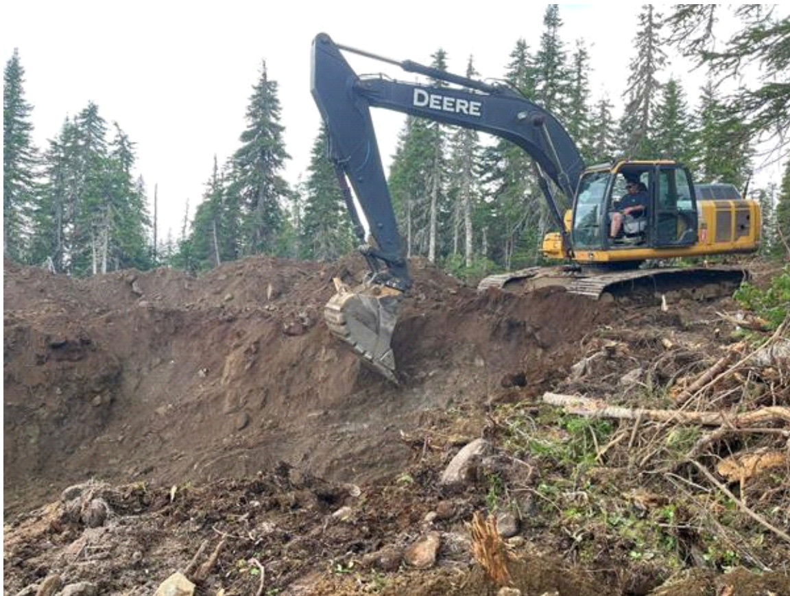
Figure 4.1: 25-tonne excavator completing a trench in the Trapper zone over the oxide layering trend.
