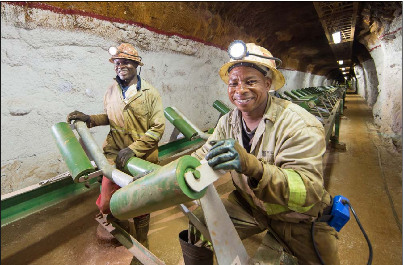
Figure 5: New rollers being installed on the 1,150-metre-level ore conveyor belt as part of the infrastructure upgrading program.
