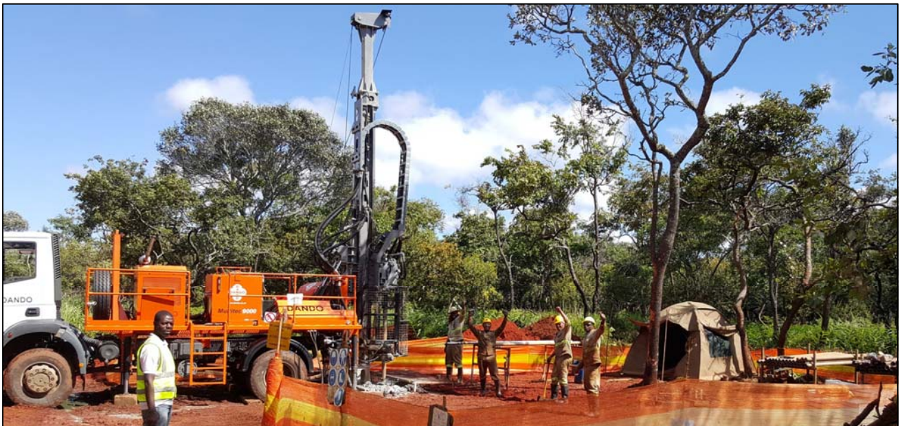
Figure 7: Drilling at Kakula West.
