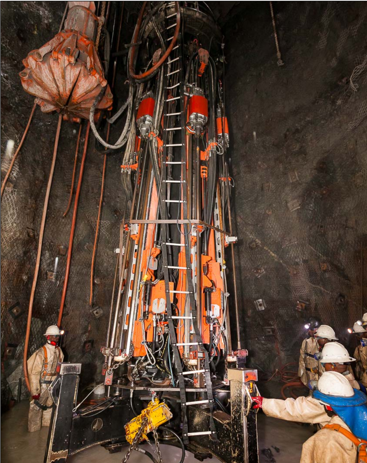
Figure 2: Members of the Platreef sinking team underground in Shaft 1, which was at a depth of 346 metres below surface on May 8, 2017.
