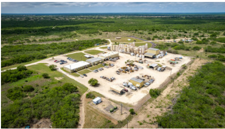
enCore Energy's Alta Mesa Plant (CNW Group/enCore Energy Corp.)
