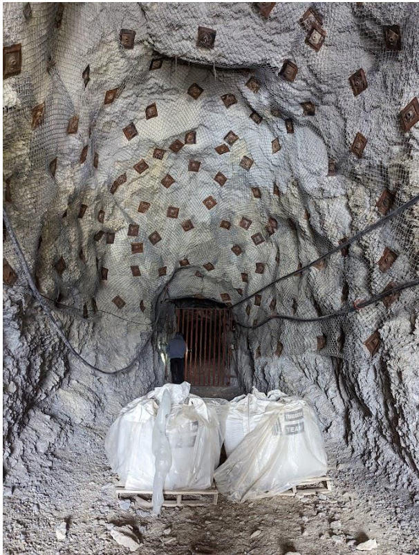
Figure 5 Supported portal area (left) and more typical unsupported underground tunnel with rails, air, power and water lines fixed to the backs (right).
