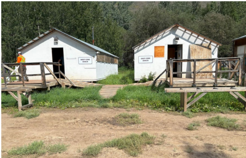
Figure 12.5 Section of the Secure Core Shed Facilities at the Coffee Gold Project
