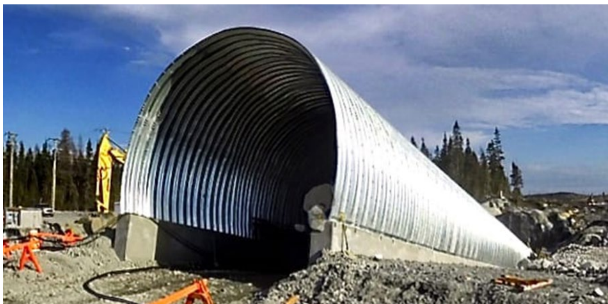
Figure 16.71: Example of a Mine Portal Culvert
