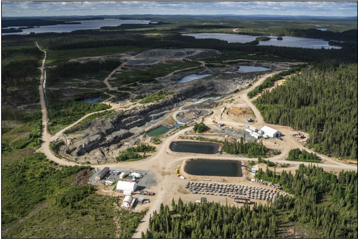
FIGURE 5.5 AERIAL VIEW LOOKING SOUTHWEST OVER THE BARRY MINE SITE AREA
