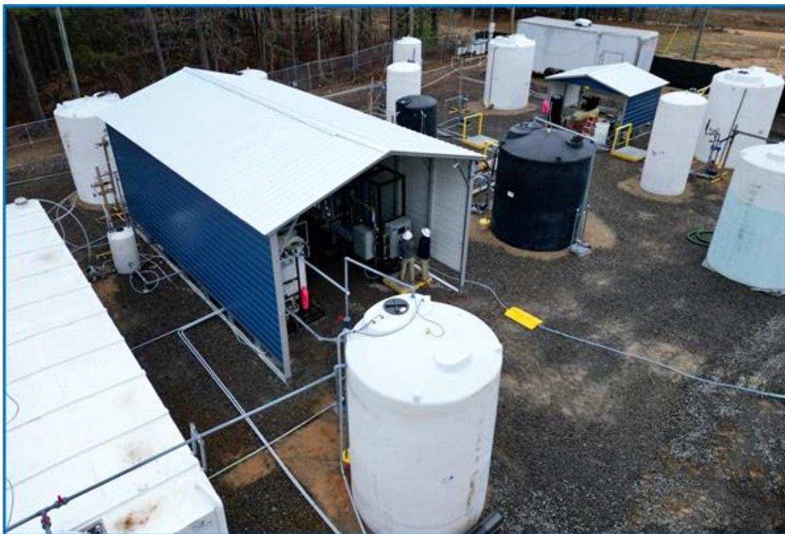
Figure 1 – Standard Lithium operators checking performance of the DLE field pilot. The larger blue and white enclosure houses the pre-treatment, filtration and DLE (LSS column) process steps.
