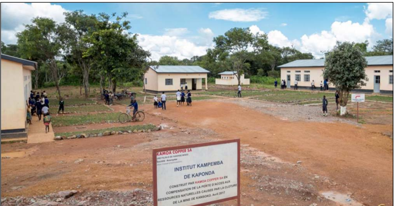
Figure 17: Upgraded buildings at the Kaponda Primary School – one of the schools constructed and furnished by Ivanhoe Mines.
