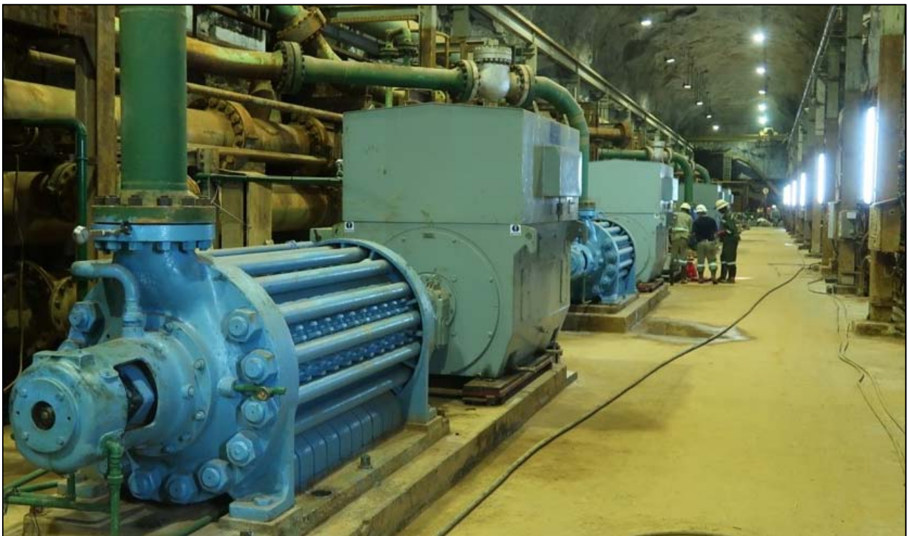
Figure 4: New high-capacity water pumps at Kipushi's 1,200-metre level.
