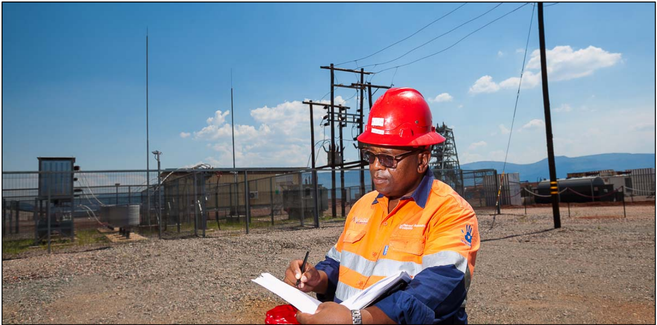
Figure 3: Eskom's 5MVA line to the Platreef Project.
